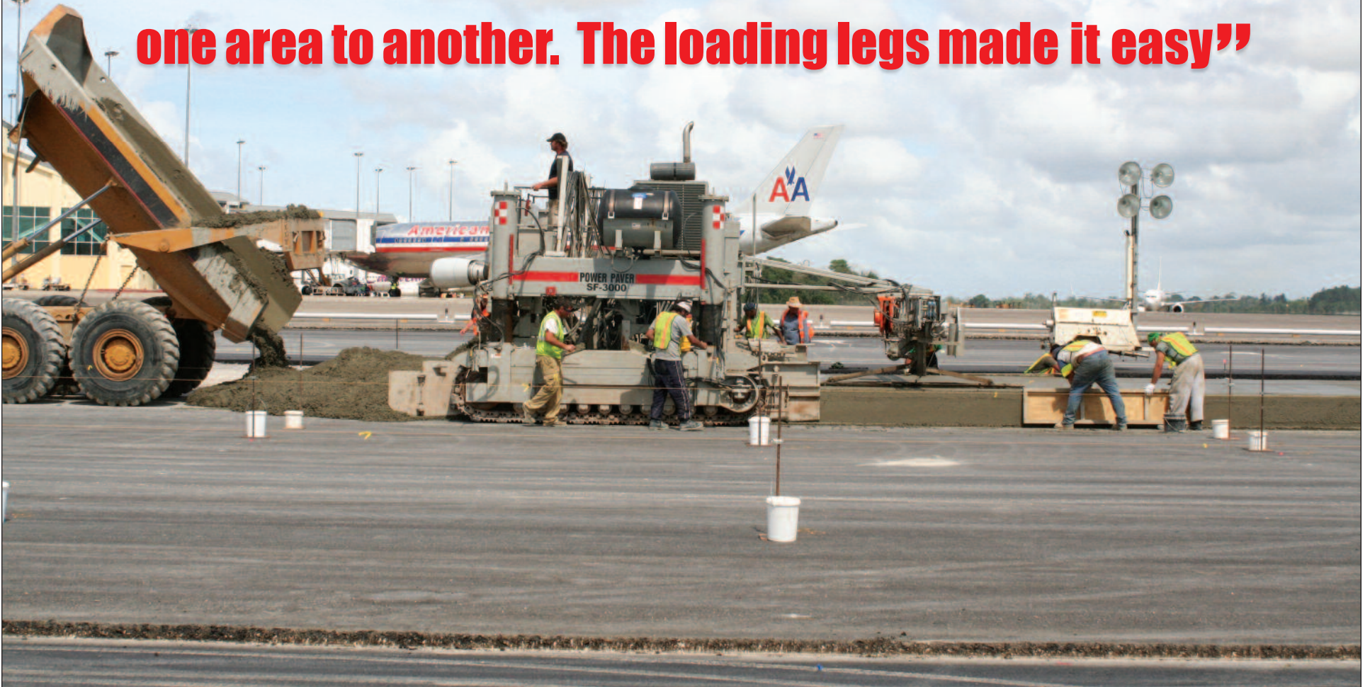
Power Pavers SF-3000 paving at Piarco International Airport in Trinidad.
