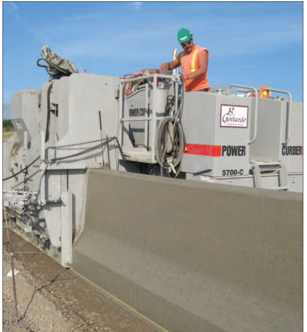
5700-C Pouring Variable Barrier in Toronto
