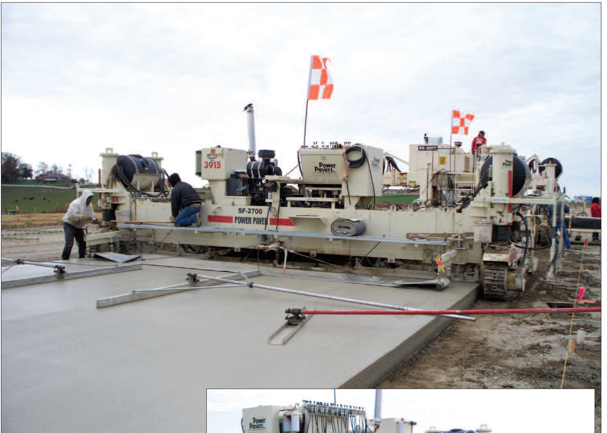
Metro Pavers SF-2700 paving 25 ft. wide on an airport runway extension.
