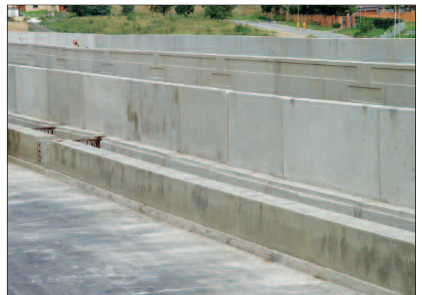
Finished pour showing both the leveling pad and conduit encasement.
