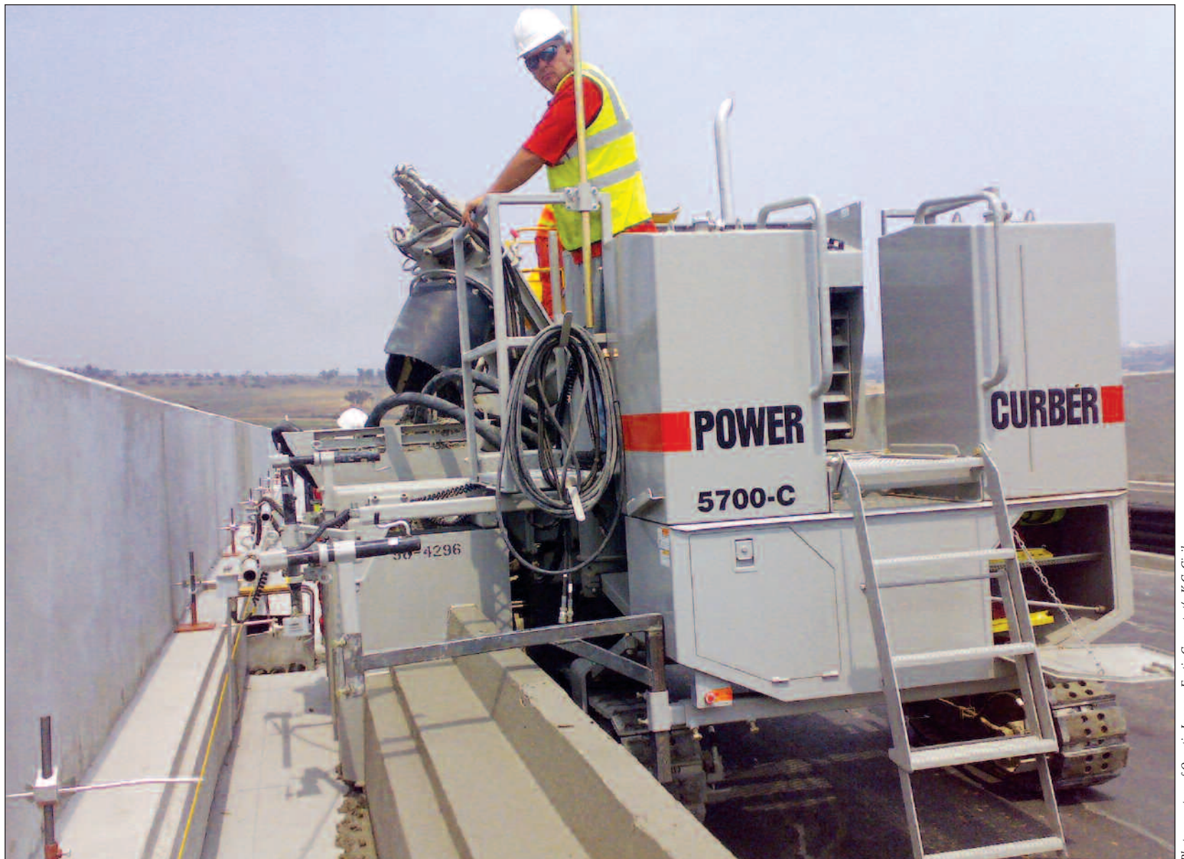
5700-C pours on viaduct deck for high speed railroad in South Africa.
