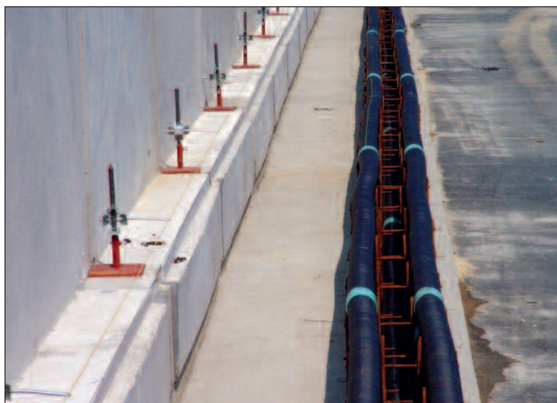
Steel baskets/conduit over which a concrete encasement was slip formed.
