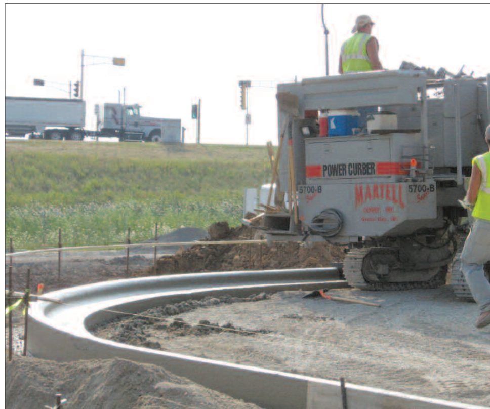
Martell crew headed toward 350,000 feet (106,750m) per year
