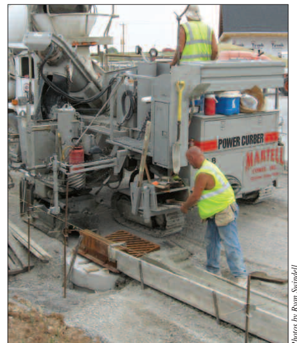
Lifting over a catch basin
