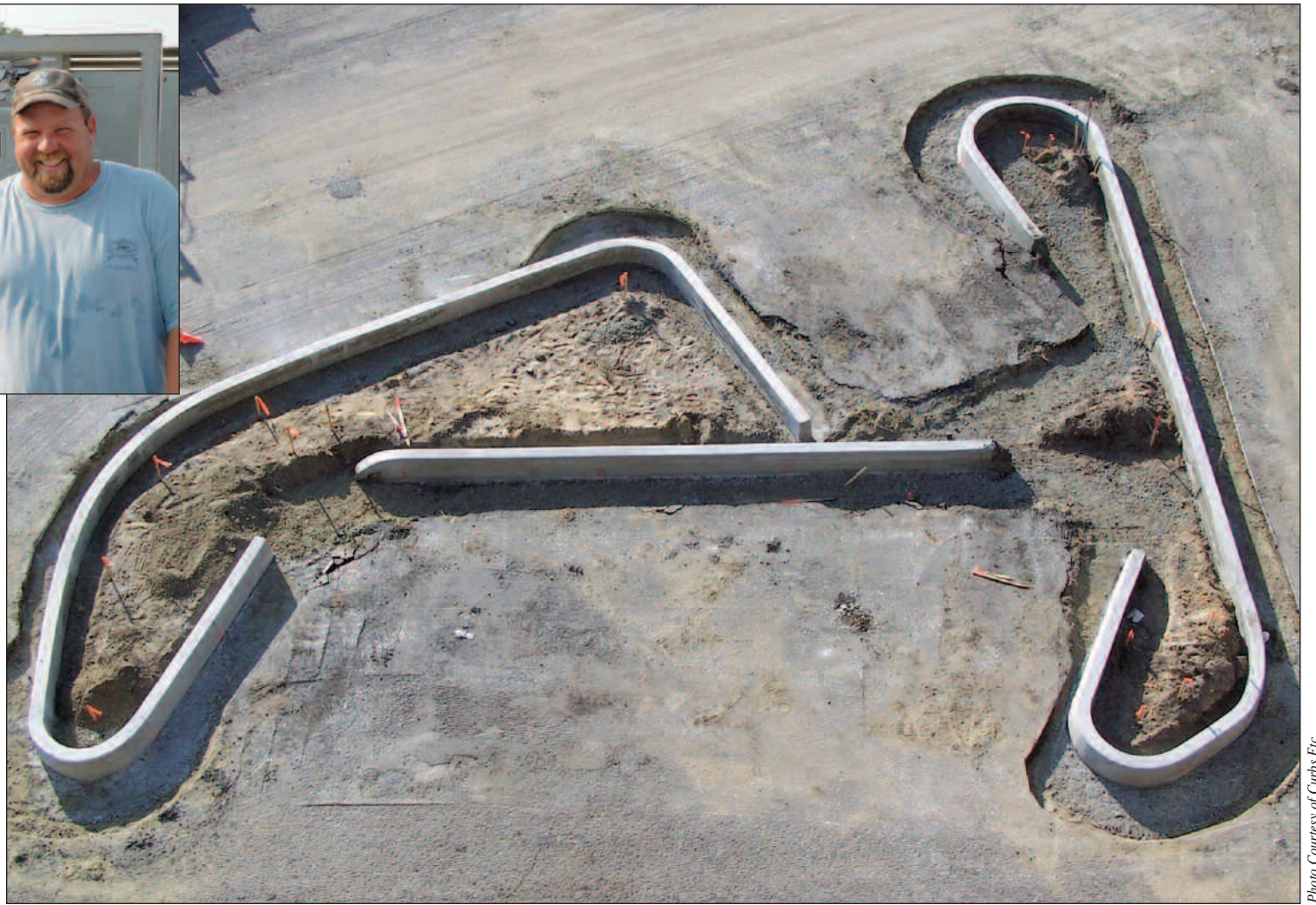
Charlie Ewing's work at a Delaware beach complex: 'The hardest part is when you start at 2.5 feet (.76m) and change to 3 (.9m), then wider,' Charlie says
