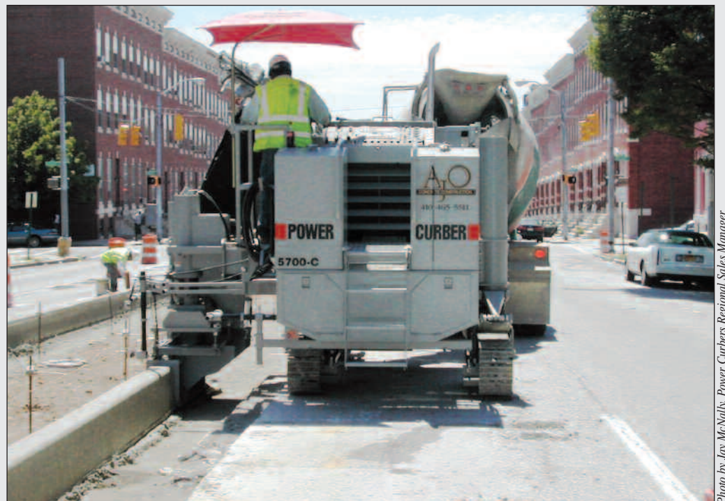
Rehab work on a city street with ready-mix truck directly in front of machine. AJO is using all 24 inches (61cm) of hydraulic side shift on the mold.
