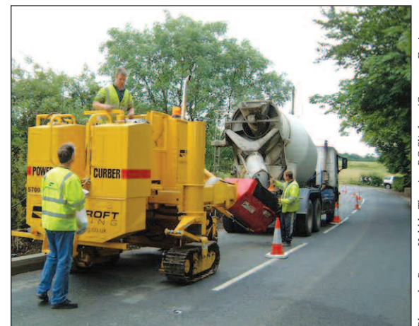
Truck lines up directly in front of curb machine
