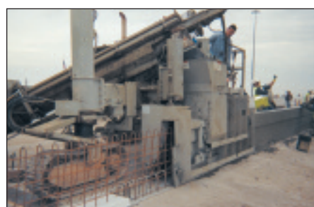
This 42-inch (106cm) parapet requires stiff concrete to hold the unsupported decorative 'lip' in place. South Coast Construction's crew poured 8,900 feet (2,714m) of the parapet with 'lip' on this job
