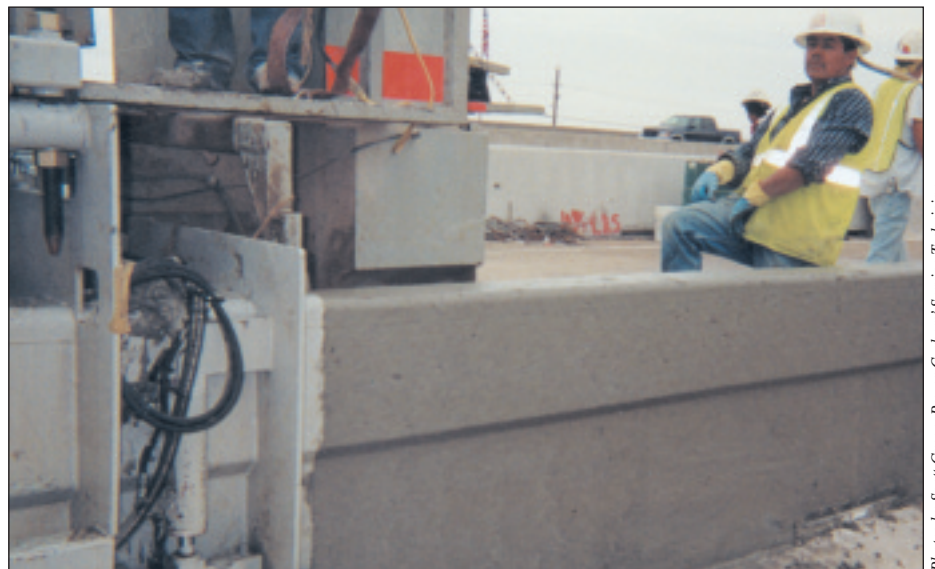
This 42-inch (106cm) parapet requires stiff concrete to hold the unsupported decorative 'lip' in place. South Coast Construction's crew poured 8,900 feet (2,714m) of the parapet with 'lip' on this job
