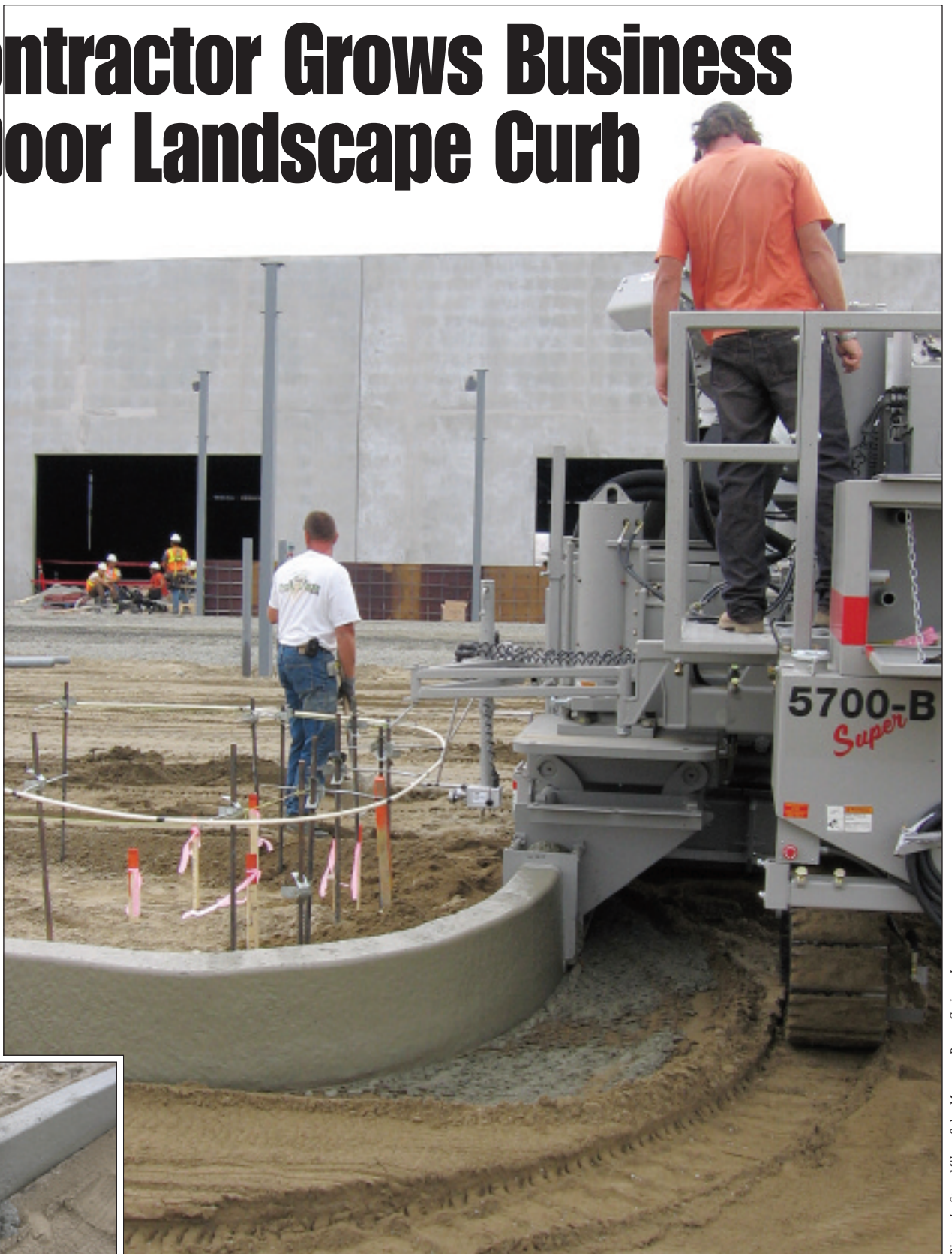
Tight radius work by Curb Appeal in Wenatchee, WA
