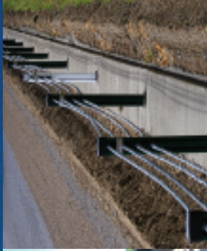
POWER CURBER Wire rope foundation and drilling
