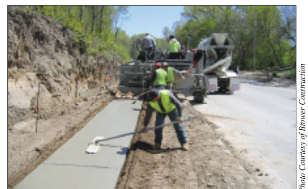
Brower Construction crew slipforming sidewalk
