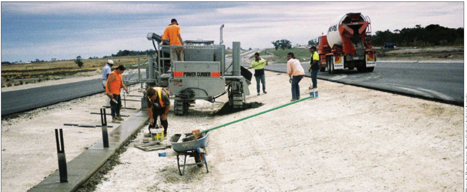
Crew knocks posts into the concrete-filled bore holes, after SUPER-B slipforms the strip. Highway safety cable will then be installed on posts. The strip prevents grass from growing under the safety cables and make road mowing easier
