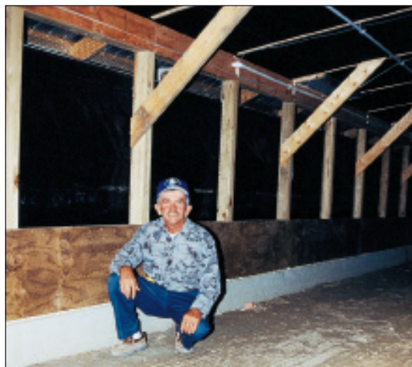
Dale Collins Sr. shows 10-inch exposed portion of 22-inch foundation wall that is slipformed in trench
