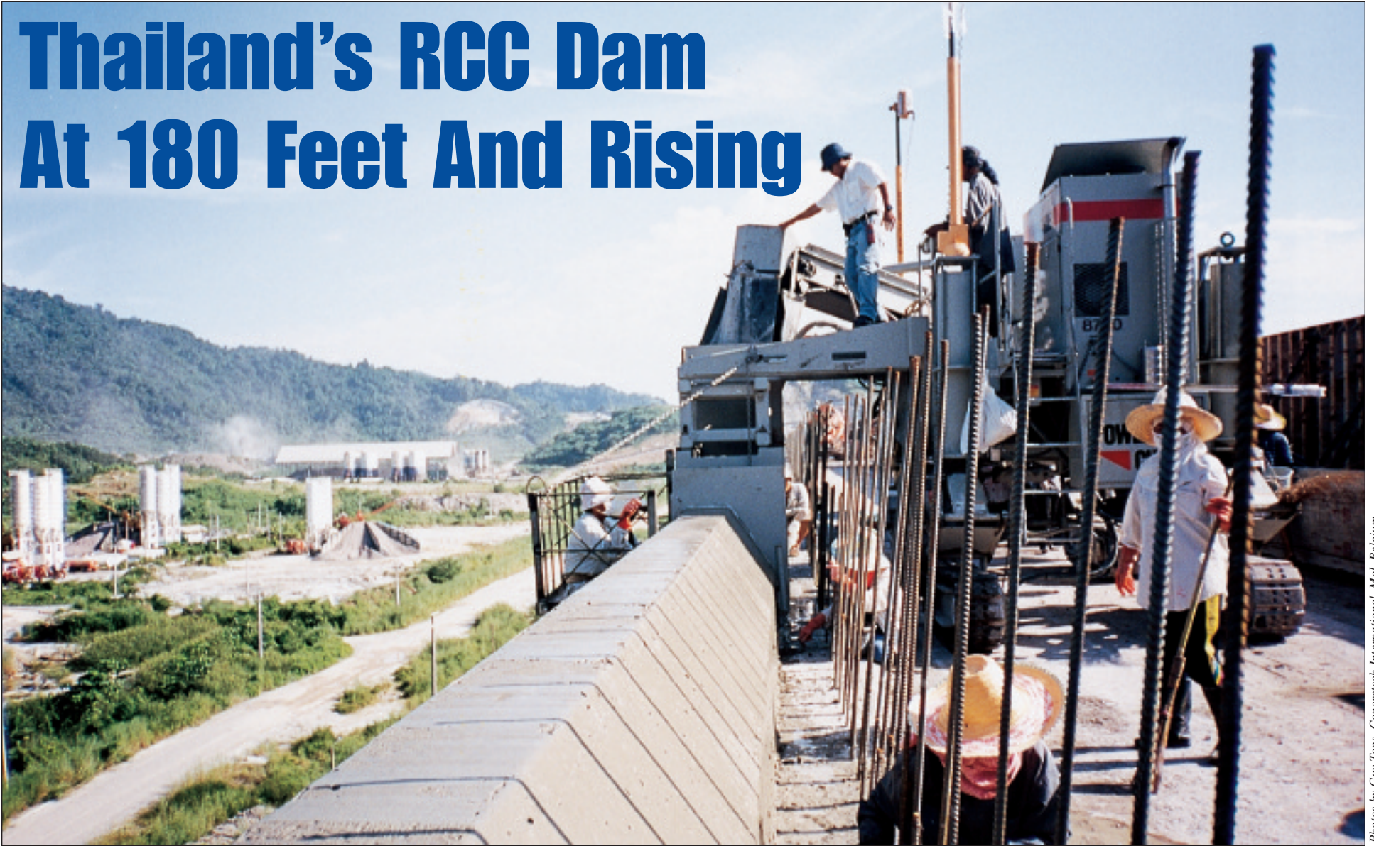
The 8700 passes over the rebar reinforcement being inserted into the upstream face of the dam
