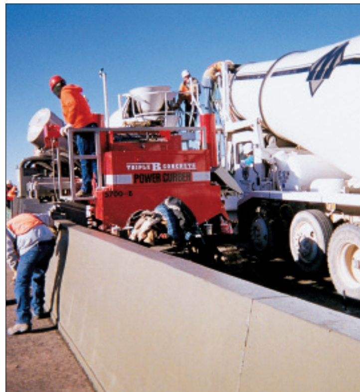
42-inch (106.6 cm) constant-slope parapet on the interchange bridge
