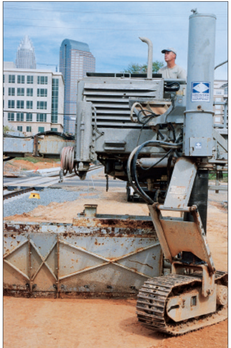
... machine being driven over center-pour mold with hopper attached
