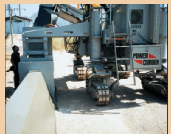
Upstream slope created by first mold
