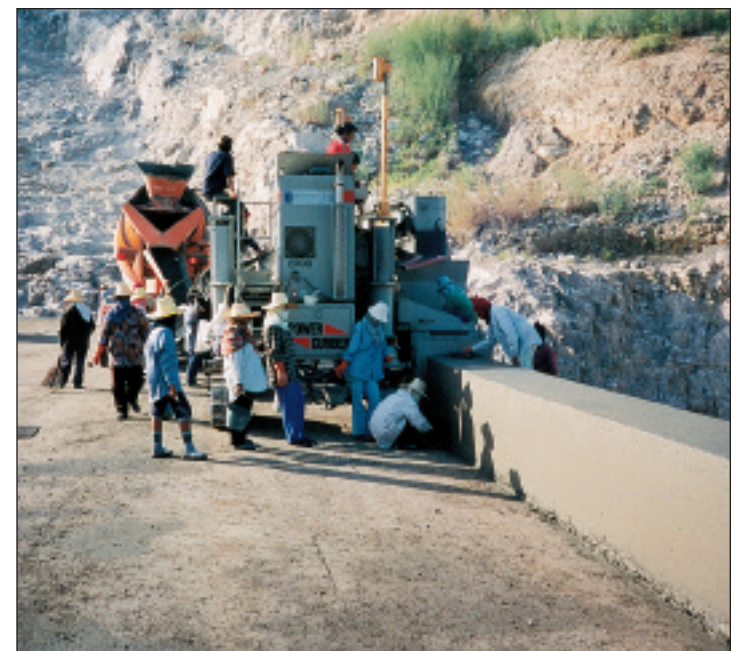
At the peak of production, the four 8700s will work simultaneously. Two machines will slipform the downstream face and the other two will slipform the upstream face. Use of the reservoir is the dam's main purpose, instead of generating electrical power, according to Teera Ngarmcroh of CCVK Joint Venture, the contractor. In these photos, the dam is about one-fourth complete
