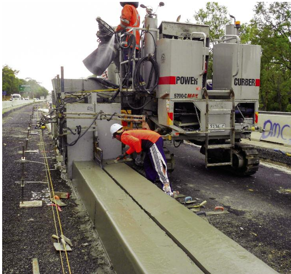
Nation Wide Slipforming in Australia slipforms a slotted drain as part of the widening of the M5 in Sydney.
