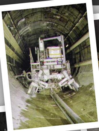
Top Left: Power Curbers engineers custom-designed the machines for the Eurotunnel project to be able to follow the curvature of the tunnel floor to pour 31 miles (50 km) of railbed.
