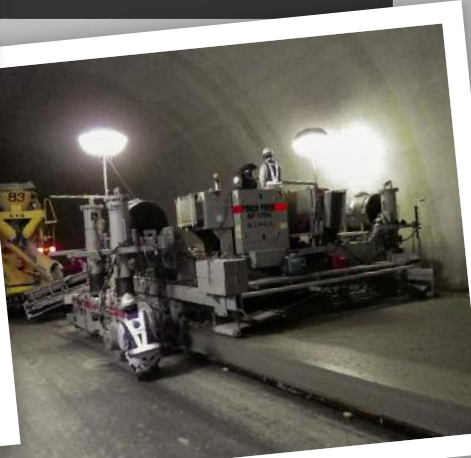
Top Left: Power Curbers engineers custom-designed the machines for the Eurotunnel project to be able to follow the curvature of the tunnel floor to pour 31 miles (50 km) of railbed.
