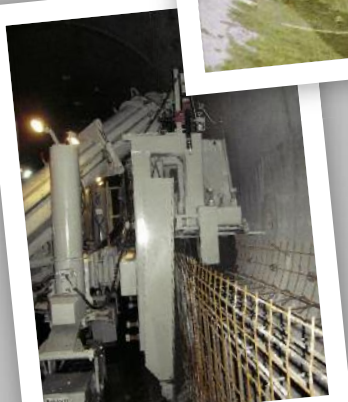
Top Left: Power Curbers engineers custom-designed the machines for the Eurotunnel project to be able to follow the curvature of the tunnel floor to pour 31 miles (50 km) of railbed.
